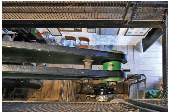
Levant beam engine. Photo Ken Geddes
